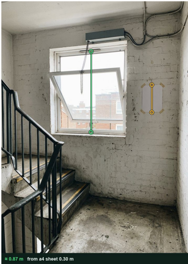
Clear frame opening height (m): measuring photo
