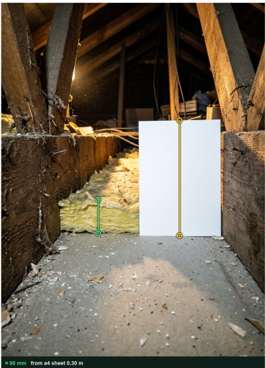
Existing insulation depth (mm): measuring photo
